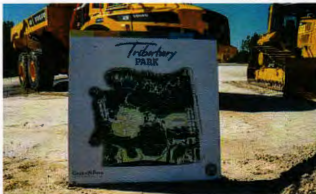
Tributary Park groundbreaking
