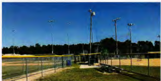
Old lighting in Yulee Sports Complex
