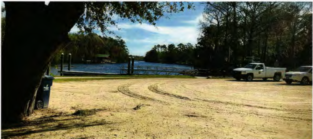
Kings Ferry Boat Ramp
