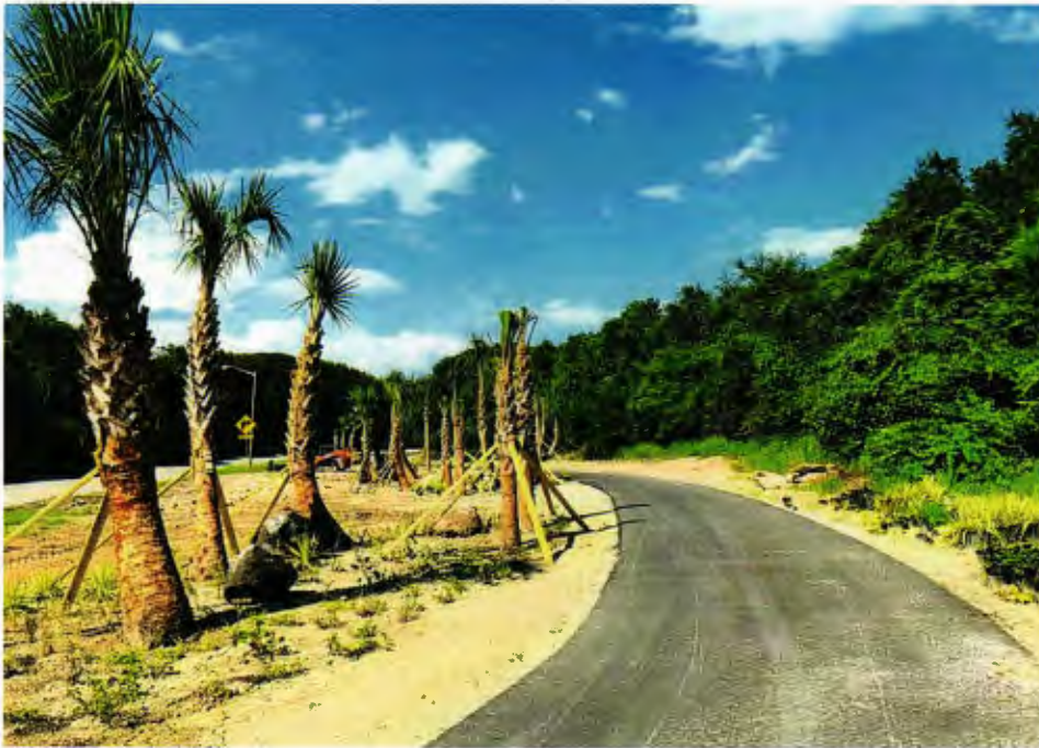
Newly constructed Amelia River to Sea Trail (ARTS) (source: https://ameliaislandliving.com/fernandinabeach/2019/09/new-amelia-river-to-sea-trail-opening/ )
