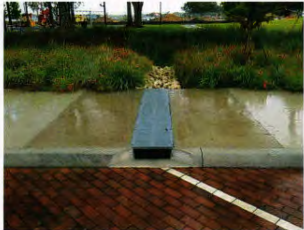
FIGURE 3.35 | Rain gardens at Kissimmee Lakefront Park
